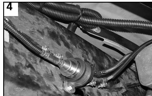
Location: Mounted to frame rail behind heater.
